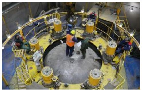
At power unit No. 1 of the Rooppur NPP being built in the People's Republic of Bangladesh, all four steam generators have been put in the planned position (by Rosatom Engineering Division ASE JSC which is the general contractor for the NPP construction). Specialists from the Energospecmontazh JSC subcontracting organisation completed assembly operations to place the steam generators in their proper positions in the reactor compartment of the power unit according to the agreed schedule.
